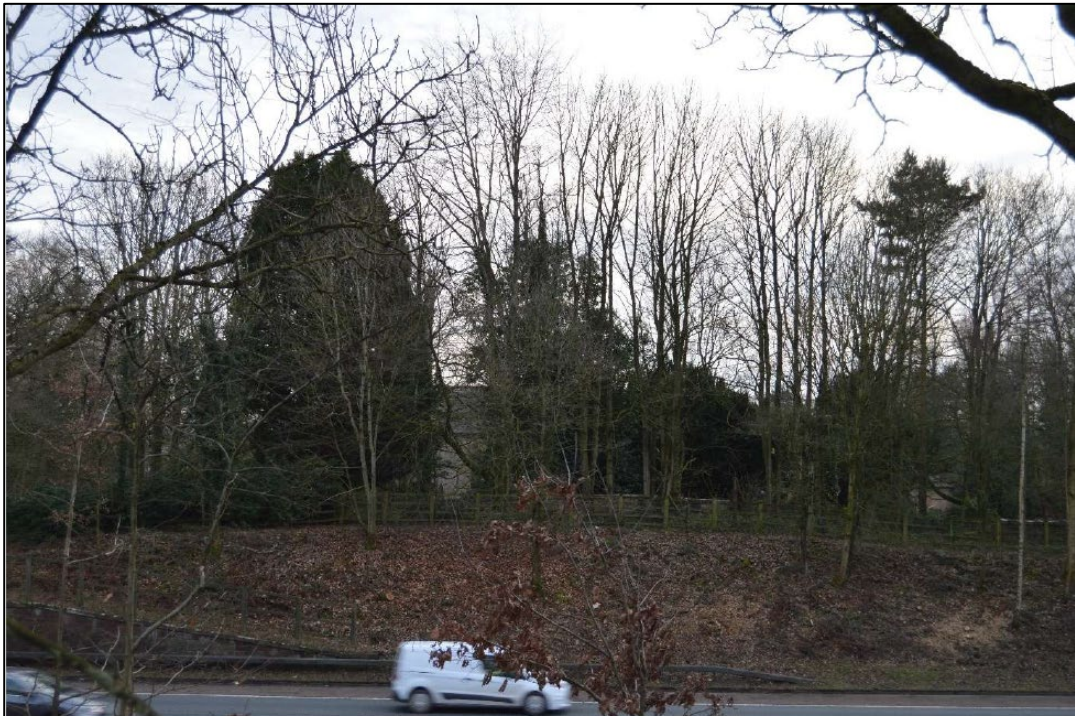
37 (125) View south-eastwards from Town Head Farm/The Steading guest House car park showing St John’s Church, Houghton within the trees. The application site lies beyond the church and is fully screened from view.
